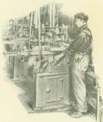
Grinding the hardened steel rollers
