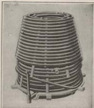
The conical-frustum arrangement of the boiler tubes
