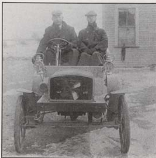
Marsh gasoline motor car, 1905-1906, Brockton, Massachusetts. Two-cylinder, 10-hp, air-cooled engine, planetary transmission, 80" wheelbase, right-hand drive, 755 lb weight. Alonzo Marsh in passenger seat.
