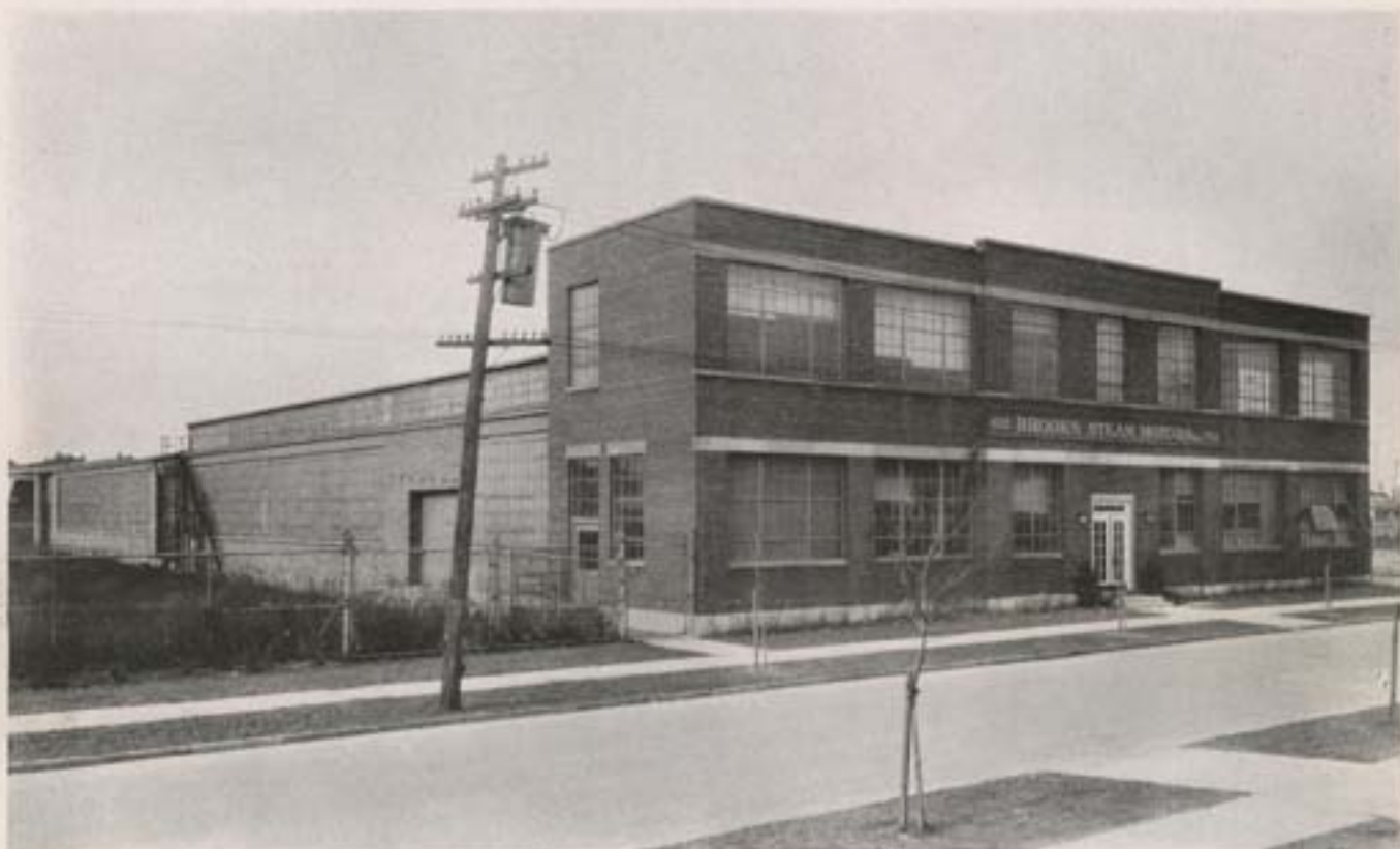
FRONT VIEW, OFFICES AND PLANT
