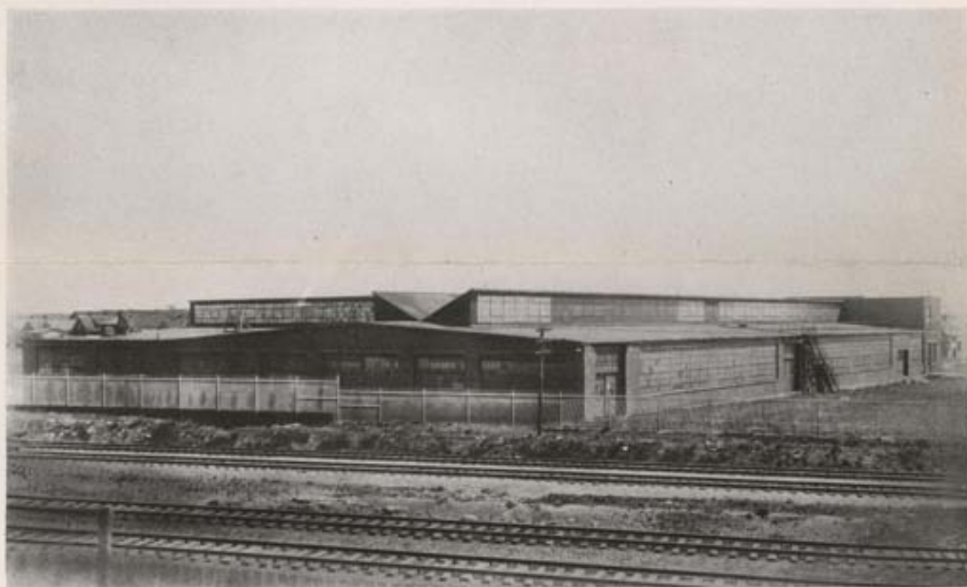
REAR VIEW OF PLANT On Lackawanna Railroad
